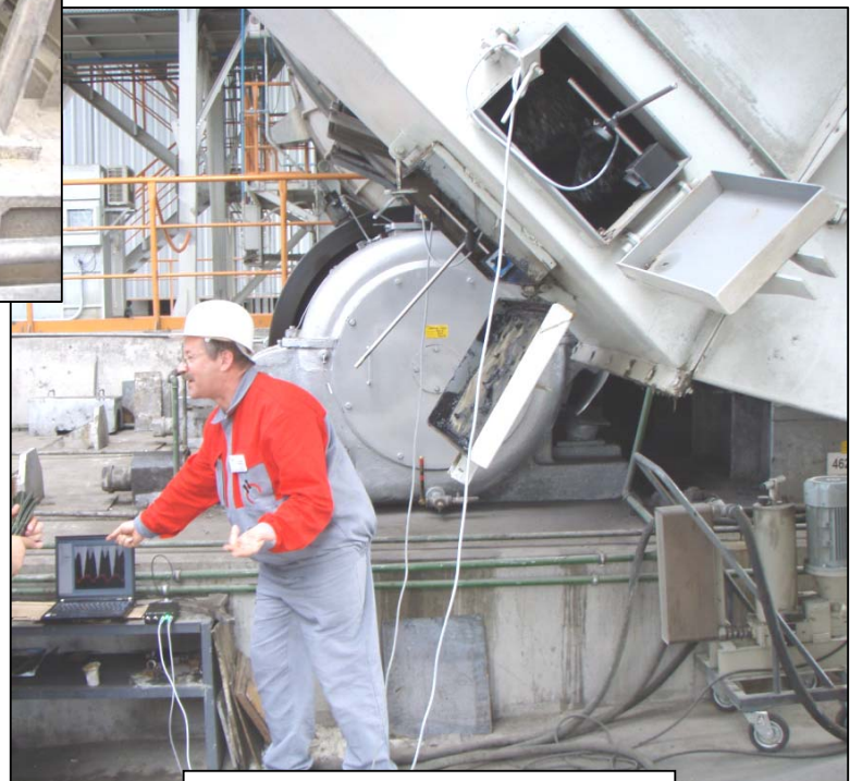
Measurement of Girth Gear Run-Out
