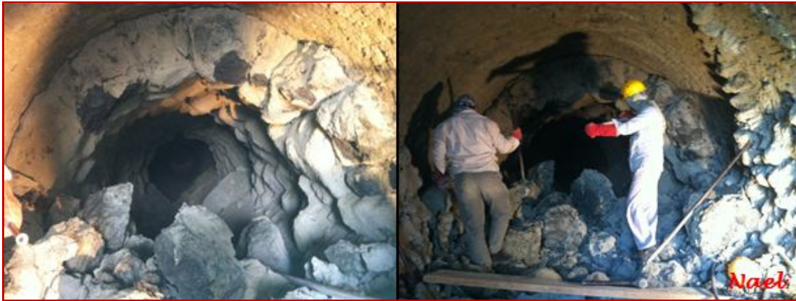
Figure-11: Kiln build-up
