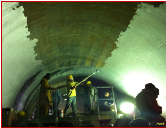
Figure-35: Kiln shell painting
