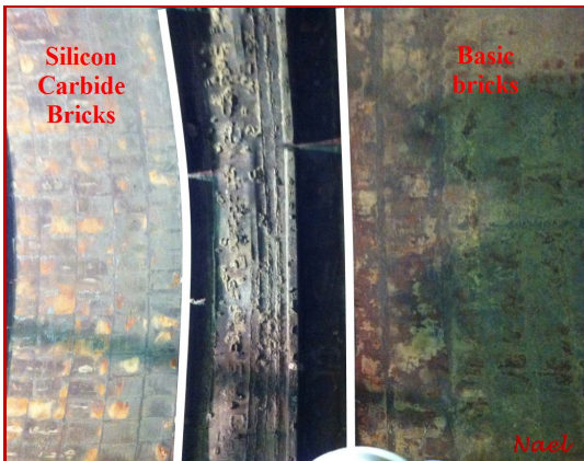
Figure-36: Kiln shell after de-lining
